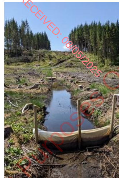
Figure 4.1: A silt trap for sediment control on a commercial forest site.
